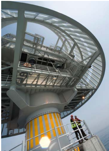
Siemens Lillgrund offshore wind park substation platform
